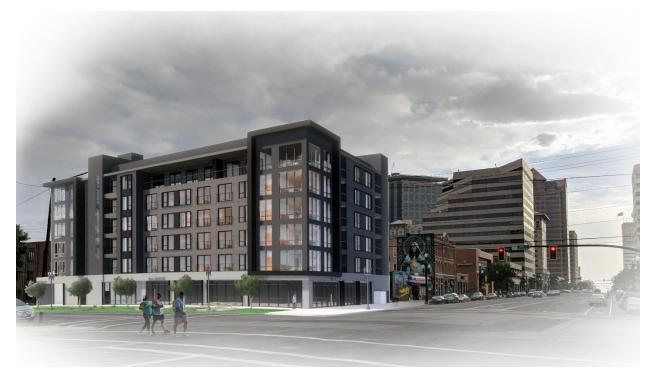
The structure is six stories in a concrete podium with stick-frame construction type. The project includes 2,300 square feet of ground floor commercial, 70 residential units, and a 7,600 square foot rooftop plaza. Some of the residential units include a small balcony of approximately 27 square feet each.
